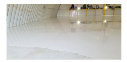
On this project, we needed extra protection for UV light, due to the large doors facing the southwest. So, we rolled on a coat of CCO-640, Stauf's exterior urethane base coat. This coat dries within 1 hour of mixing and applying with a short nap roller. Once dried, the surface was screened again with an 80 grit screen and tacked with acetone to make sure it was completely clean.
