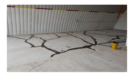
The floor was then primed with a 2 component water based epoxy, Stauf's EHS-265. This coat has a 45 minute working time once mixed, and can be walked on in 2 hours. It will penetrate deep into the concrete, giving all coatings that follow the most extreme bond possible. It is white when applied, but will dry clear. After applying this coat, there is no need to sand the surface. At this point, the surface will be clean and ready for the next coat in the process.
