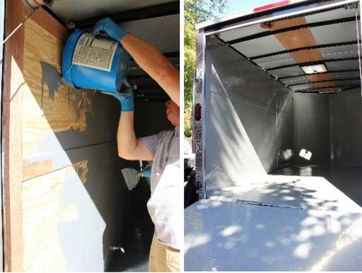
To give a smooth surface, the walls were then sanded with 120 grit sand paper using a hand sander, and a buffer with a 180 grit used screen was used on the floor. Once sanding was finished, everything was power vacuumed and then tacked off with damp rag of acetone to remove remaining dust before the next coat was applied.
